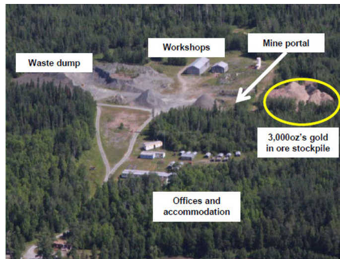
Figure 4: Aerial photograph showing surface infrastructure at Cameron
